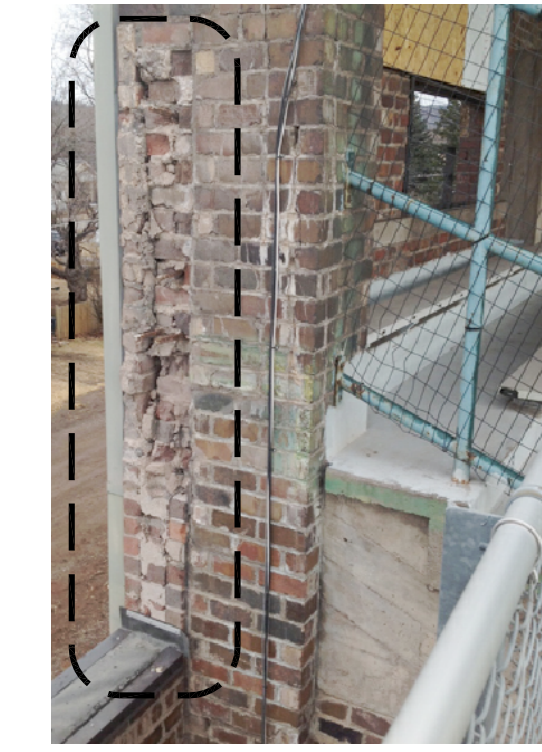
GRANDSTAND BRICK PIER CONDITION, GRID G.1G. REFER TO 3/A2.1 FOR NOTES. GRID G.3G SIMILAR.
