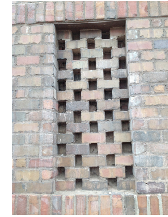
TYPICAL BRICK RECESS
