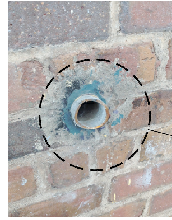
WALL-MOUNTED RAIL REMOVAL AT TWO LOCATIONS.
